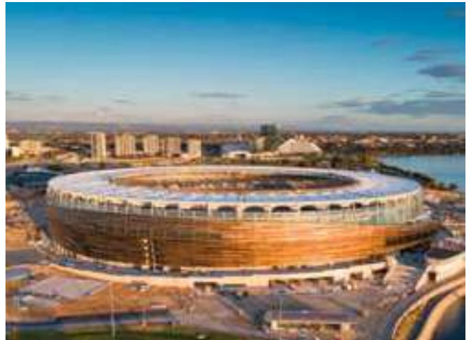
Perth Stadium - Perth (Australia)
